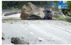
Rock fall on a motorway in Austria as a result of no mitigation measures
