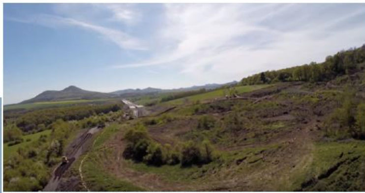
Limestone landslides completely destroyed the Motorway D8 (Zagreb – Šibenik) before opening to traffic.
