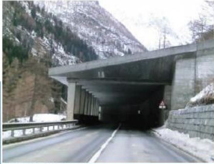
Avalanche protection by the concrete gallery
