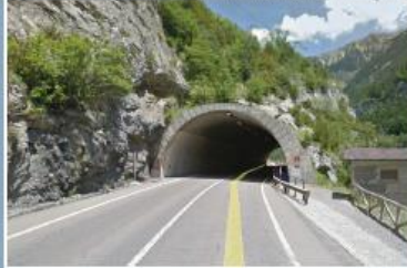
Tunnel structure protecting road against landslide or rock fall
