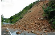
Massive landslide from an unprotected slope
