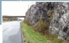
Unprotected rock cut very close to the road
