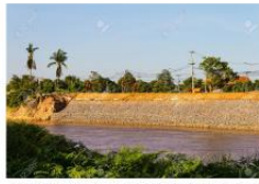
Construction of mesh stone walls to prevent water erosion
