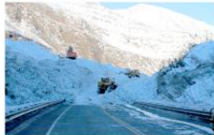
Avalanche damaging and closing a road
