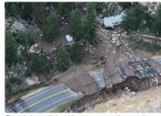
Road demolished by river erosion and simultaneously by mud from the transversal valley
