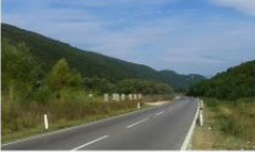
Non-resistant surface materials are vulnerable
