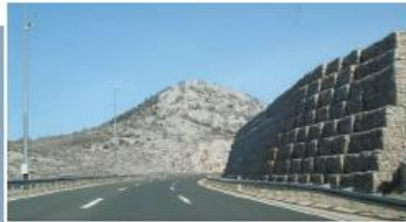
Protection against strong wind (Croatia railway)
