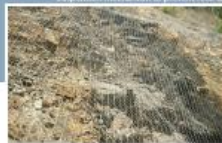
Suspension mechanism to prevent rock fall
