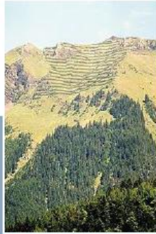
Forest and structures to protect against avalanches
