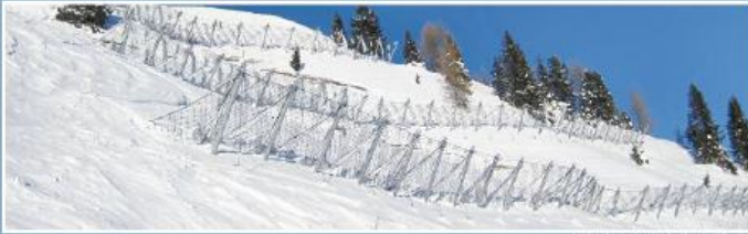
Avalanche protection by the steel bracing
