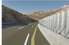
Wind protection on the right side of road (Croatia)
