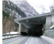
Avalanche protection by the concrete gallery
