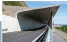
Effective protection against landslides
