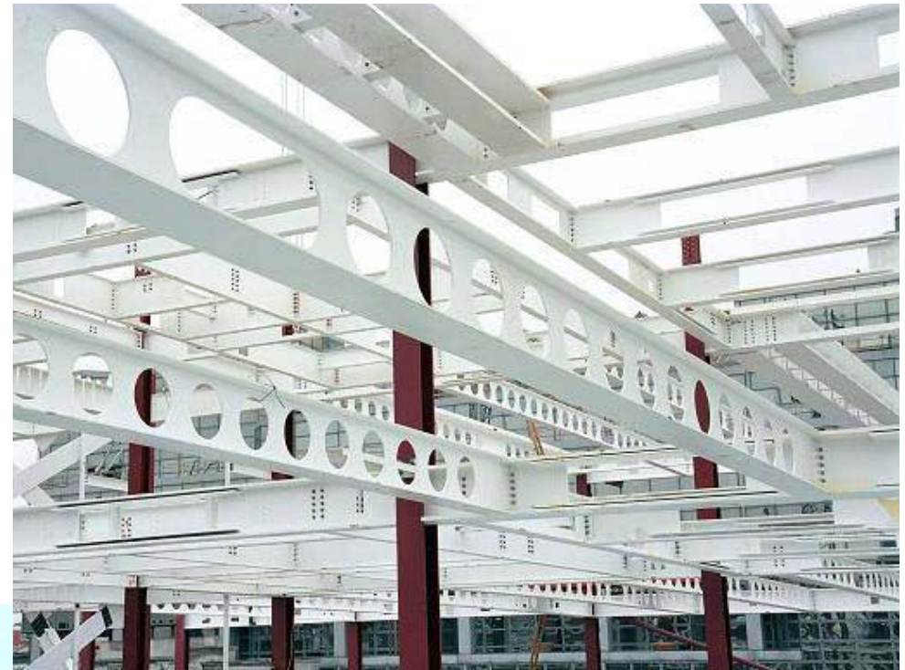
Fabricated beams with variety of shapes of openings
