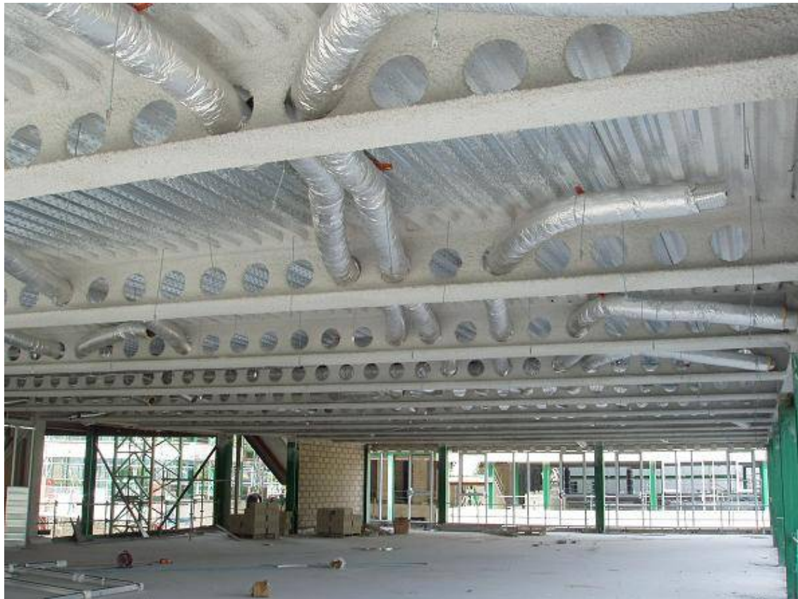
Cellular beams with regular openings for services
