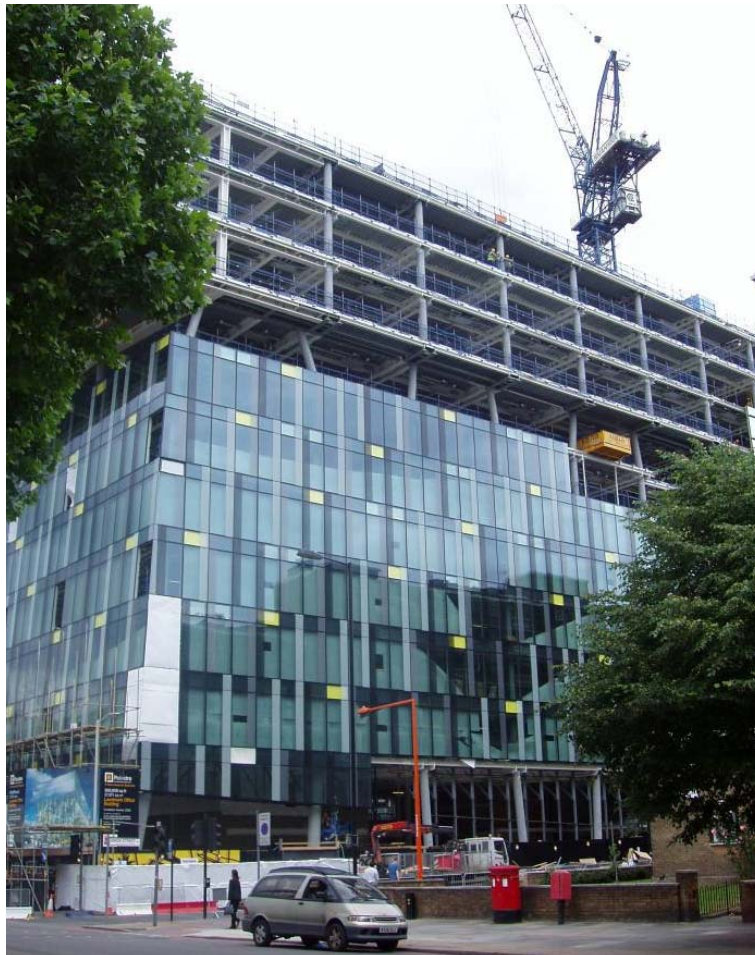
During construction, showing steel framework and fully glazed facade
