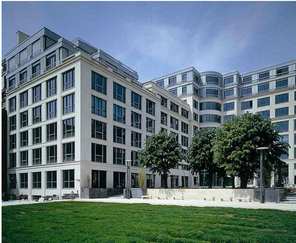
Completed building showing the new façade
