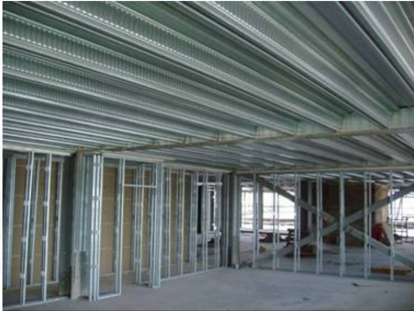
Integrated beams with deep decking
