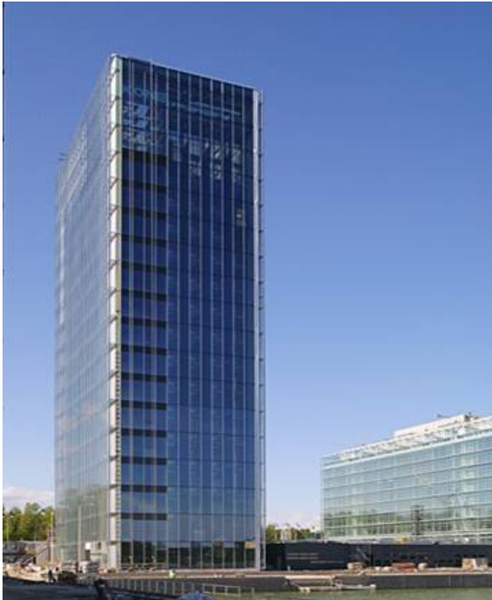
Double façade in the Kone Building, Finland
