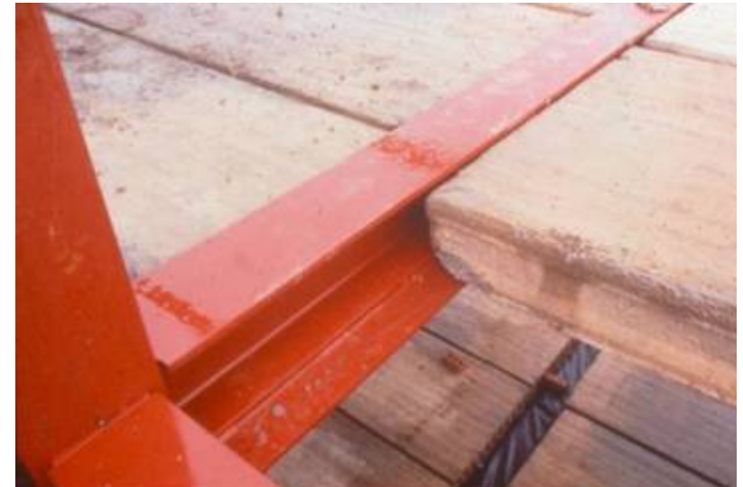
Integrated beams supporting precast concrete slabs
