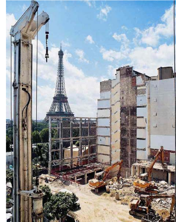
Demolition stage of the original concrete frame
