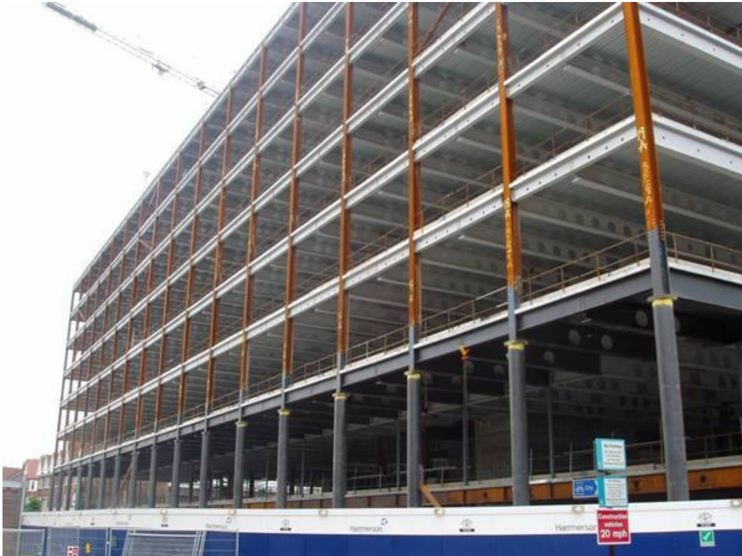
Tubular columns exposed for fire resistance
