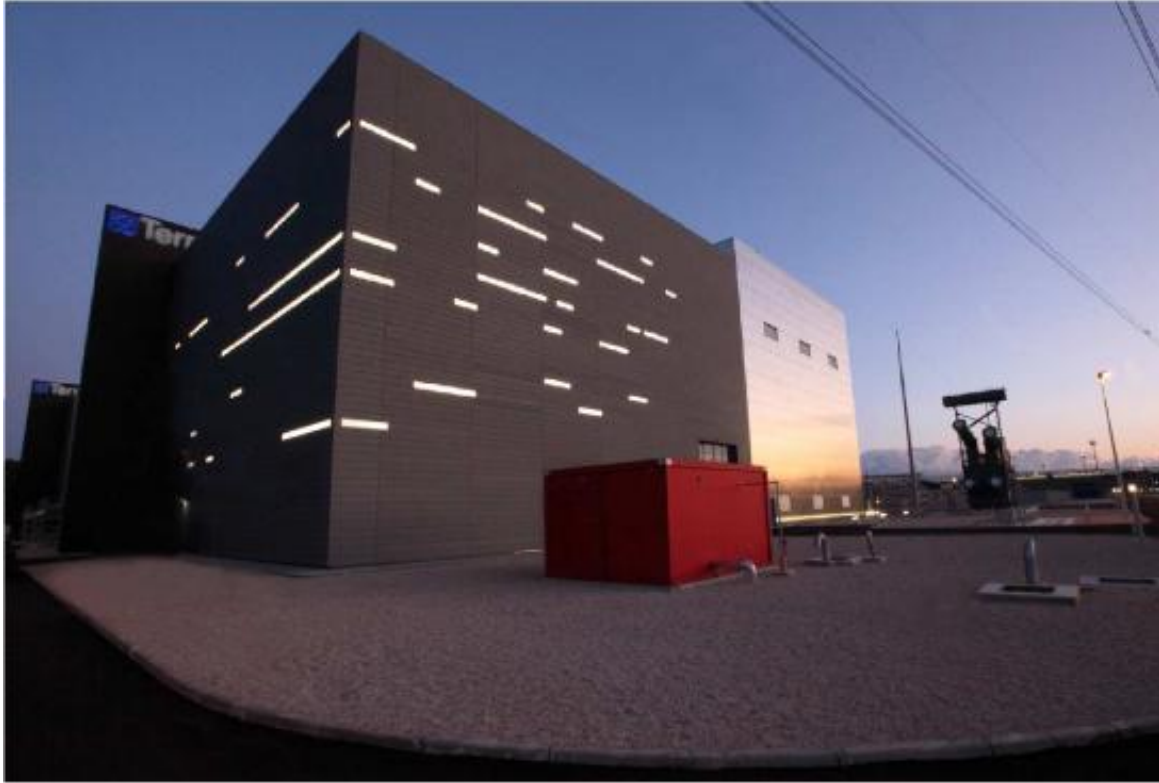
picture 4 – Example of a converter station
