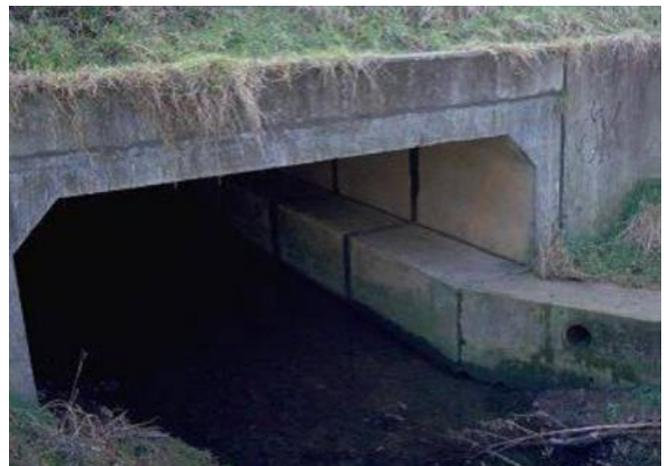
Figure 21: Potential Design for a Culvert for Amphibians, Reptiles and other Small Animals
