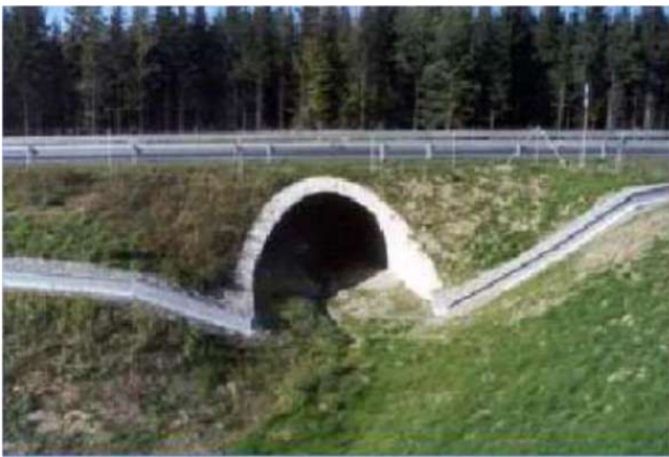
Arch culvert with fence for large mammals and lipped wall for amphibians (FHWA/US DOT, 2002)
