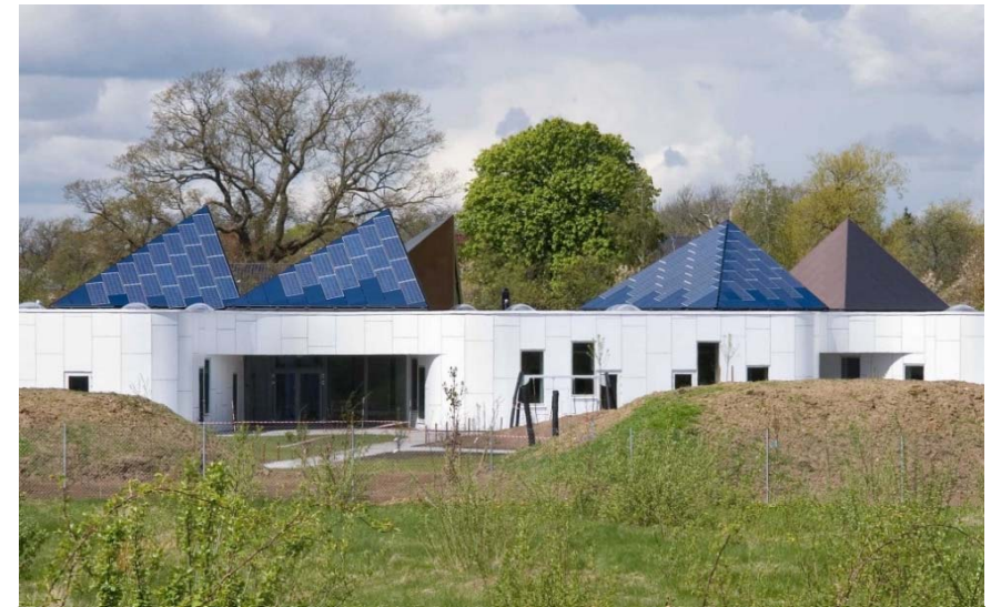
Solar panels on the roof © Cebra
