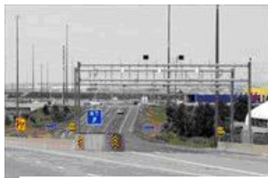
An example of a fully automated system showing the access ramp and overhead gantry with detector beacons.
