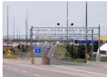
An example of a fully automated system showing the access ramp and overhead gantry with detector beacons.
