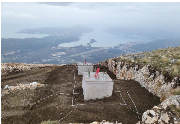
Grounding system installation for towers S17 to S19
