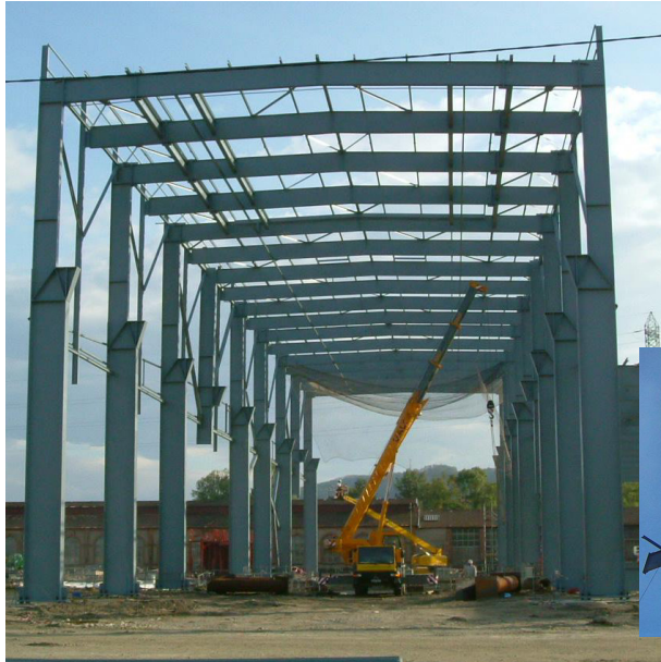
Typical heavy industrial building, with a height of 22 m and spans of up to 23 m.
