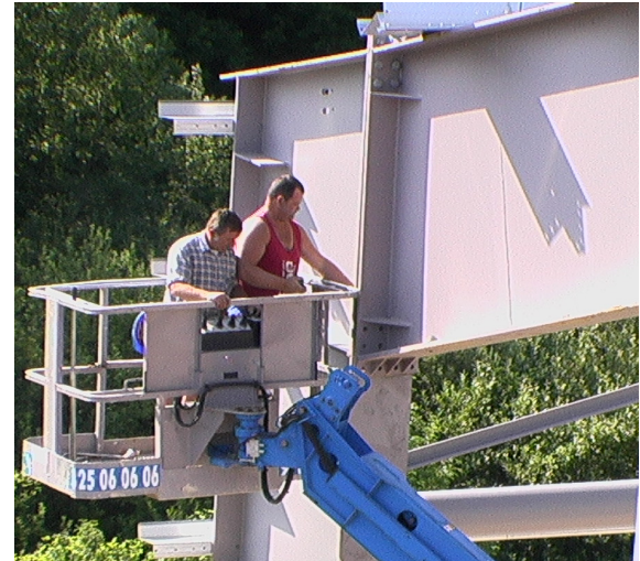
General view of the structure during erection
