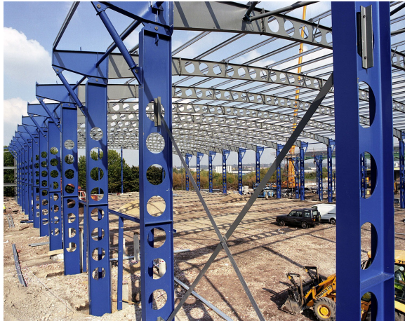
Innovative moment-resisting connections in an industrial building
