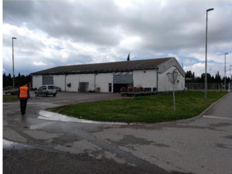
Figure 46 TGD Cargo Terminal Building
