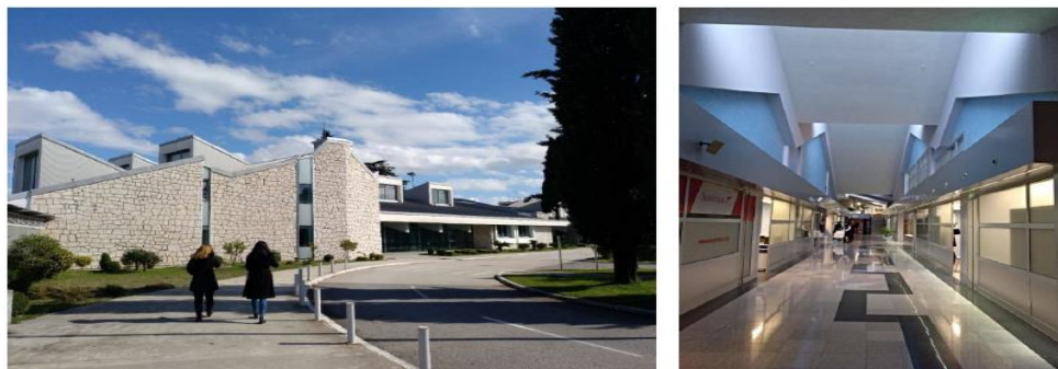
Figure 45 TGD Administrative Building
