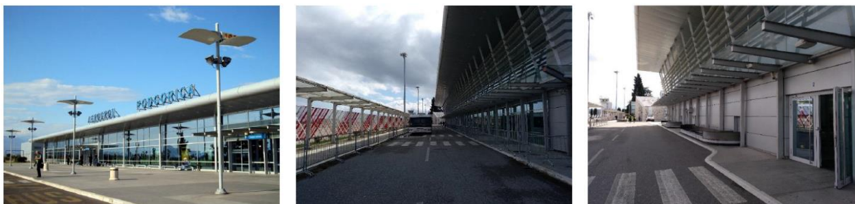
Figure 41 TGD landside façade, departures façade, arrivals façade of the passenger terminal
