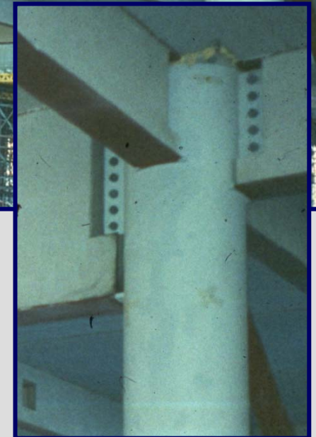
Load introduction with gusset plates
