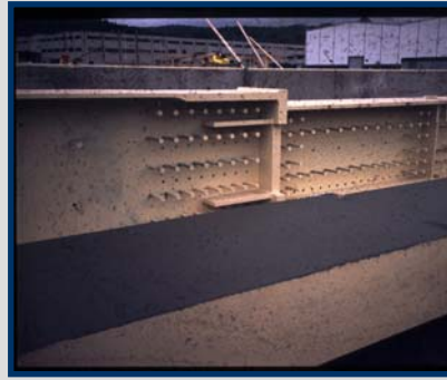
partially concrete encased sections
