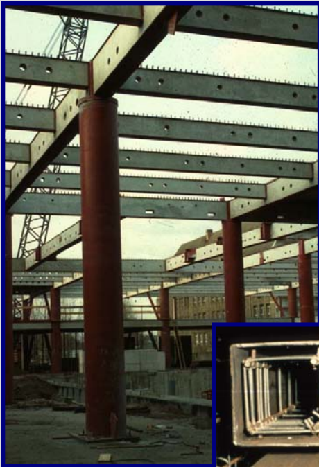
concrete filled hollow sections
