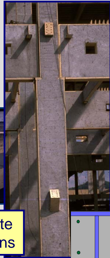
concrete encased sections
