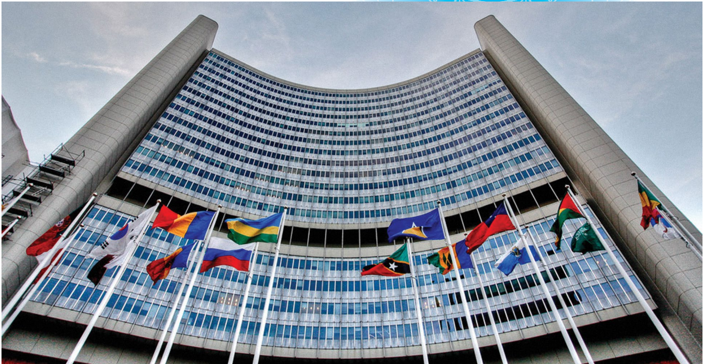
International Atomic Energy Agency headquarters in Vienna
