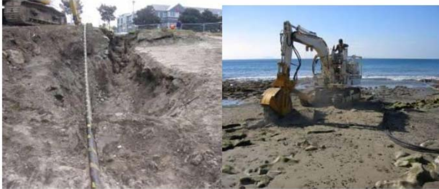
pic.29. trench example
