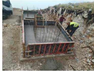
Figure 10-6: Casting of S7 foundation slab and placement of reinforcement at S8
