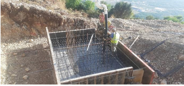
Figure 10-6: Casting of S7 foundation slab and placement of reinforcement at S8
