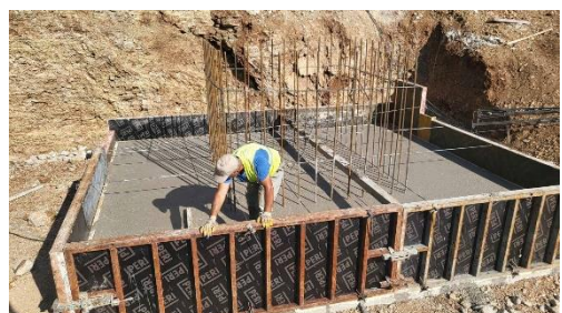
Figure 10-4: S5 and S6 after excavation and placement of concrete underlay
