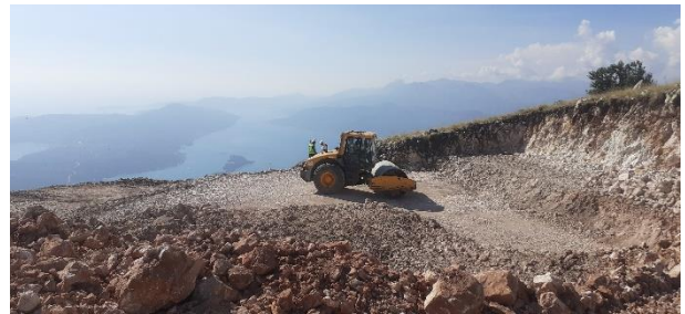
Figure 10-8: Excavations at S19 and the top station, compaction of soil at the top station
