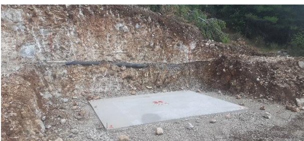
Figure 10-4: S5 and S6 after excavation and placement of concrete underlay
