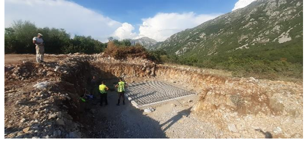
Figure 10-6: Casting of S7 foundation slab and placement of reinforcement at S8
