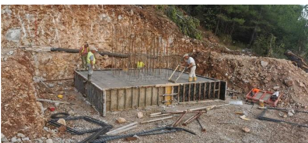
Figure 10-5: S5 and S6 after casting
