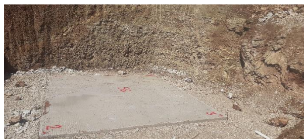
Figure 10-4: S5 and S6 after excavation and placement of concrete underlay
