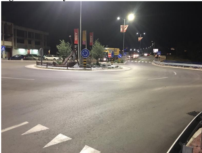
Figure 2.1: Newly constructed roundabout near the survey location
