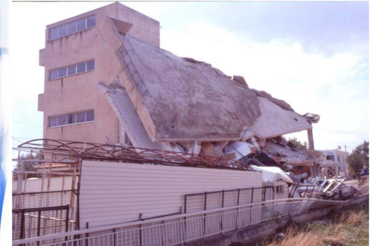
Collapse of building due to its torsional response about a stiff shaft at the corner (Athens, 1999 earthquake).
