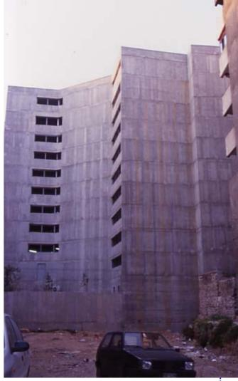
Strong column/weak beam capacity design not required in wall- or EUROCODES wall-equivalent dual systems (>50% of seismic base shear in walls)
