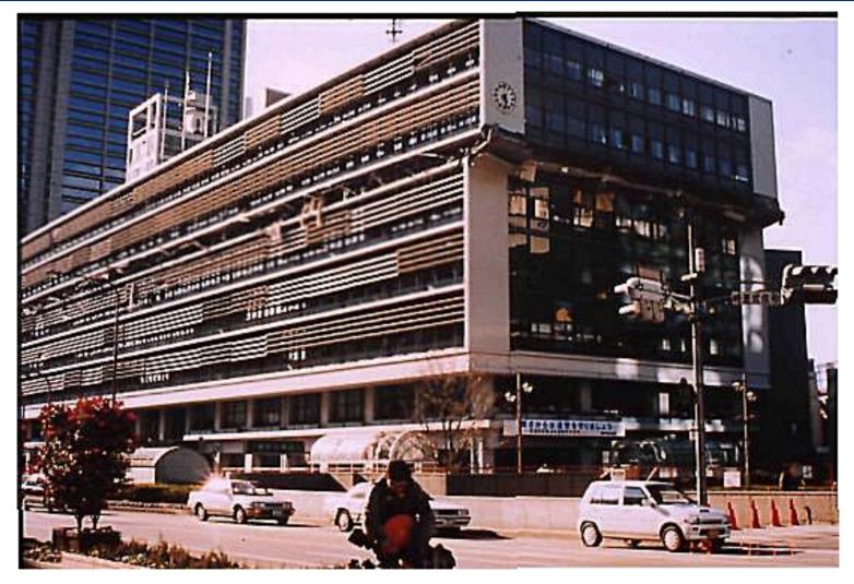
Collapse of intermediate storeys w/ reduced stiffness Kobe (JP) 1995.
