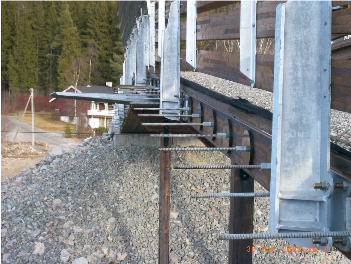
Bridge across railway, Oslo
