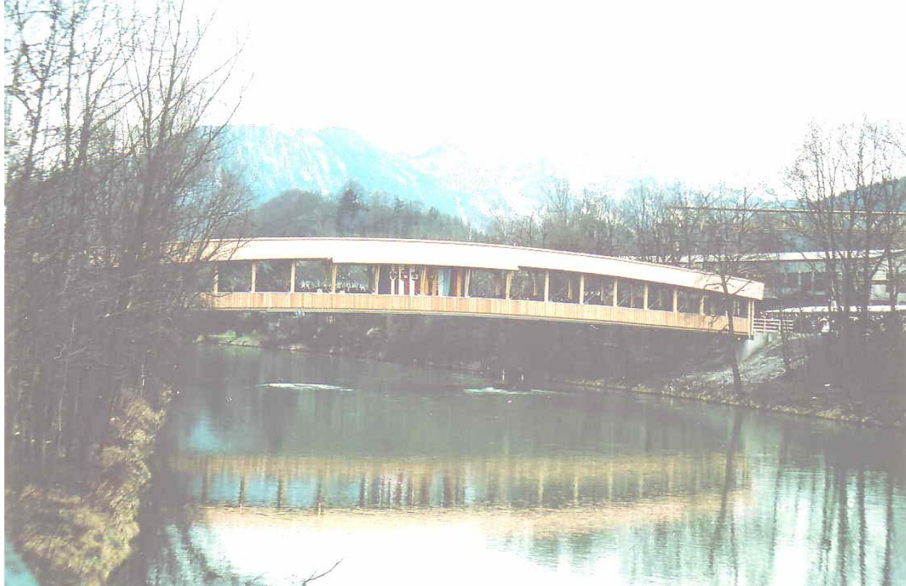
Bridge over river Saalach Bavaria - Salzburg, 70m span
