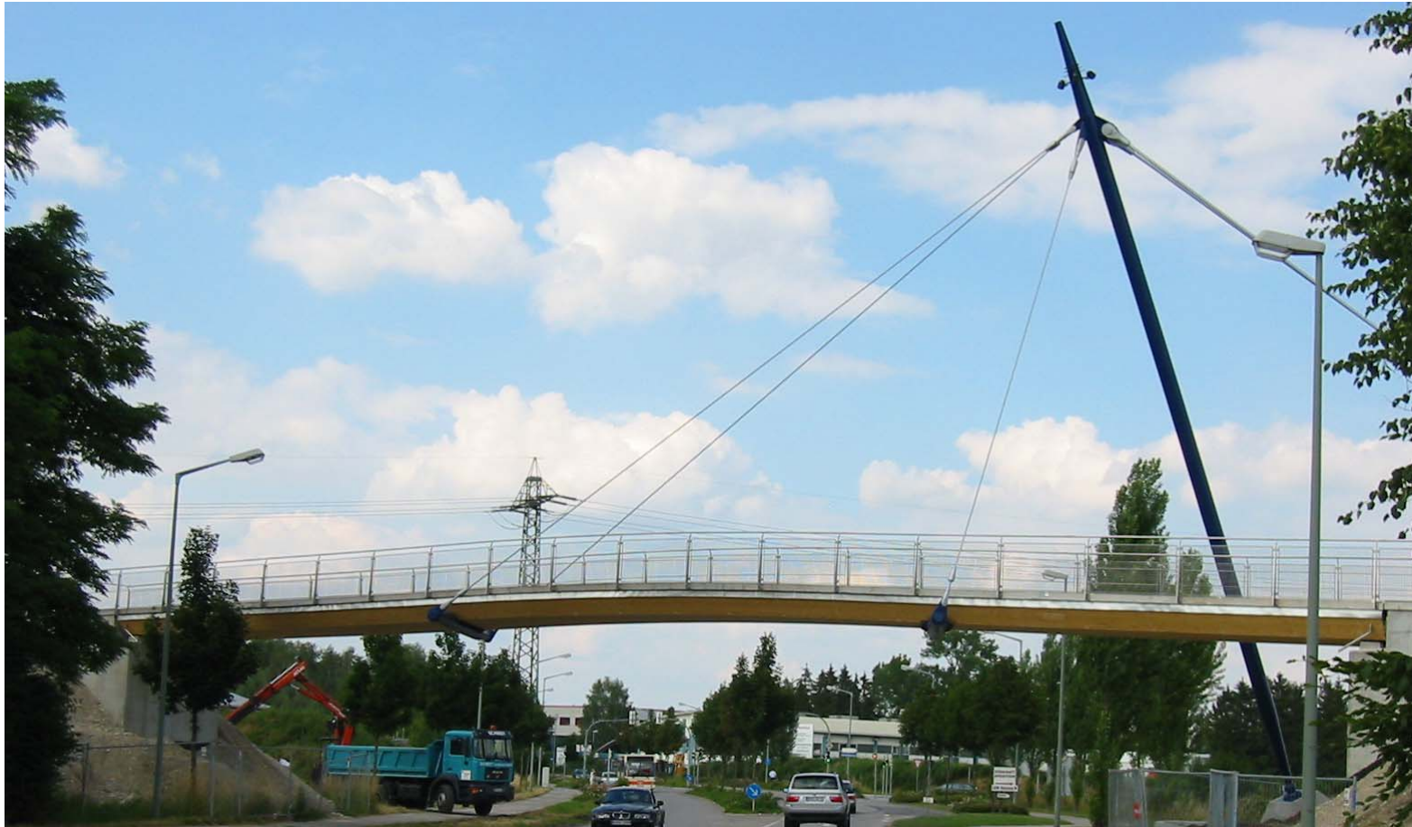
Bridge in Karlsfeld near Munich
