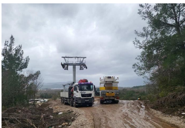
Towers S2 and S3
