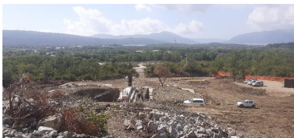
Figure 10-1: The bottom station
